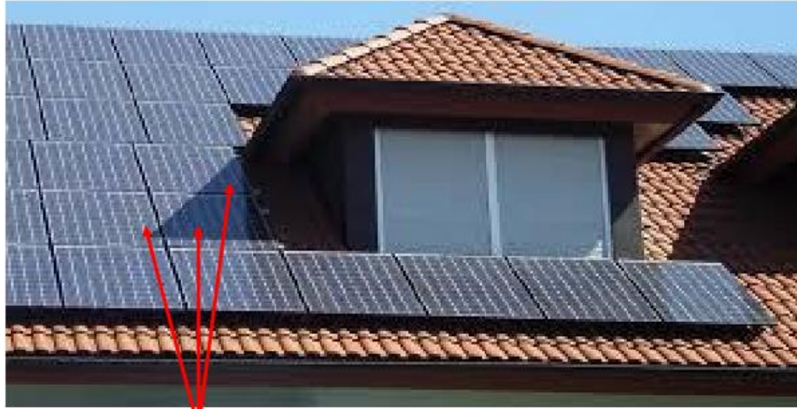
Only 3 Modules are shaded, in need for optimization
